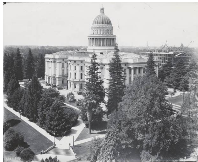
Capitol Building, circa 1924. Courtesy of the California State Library
