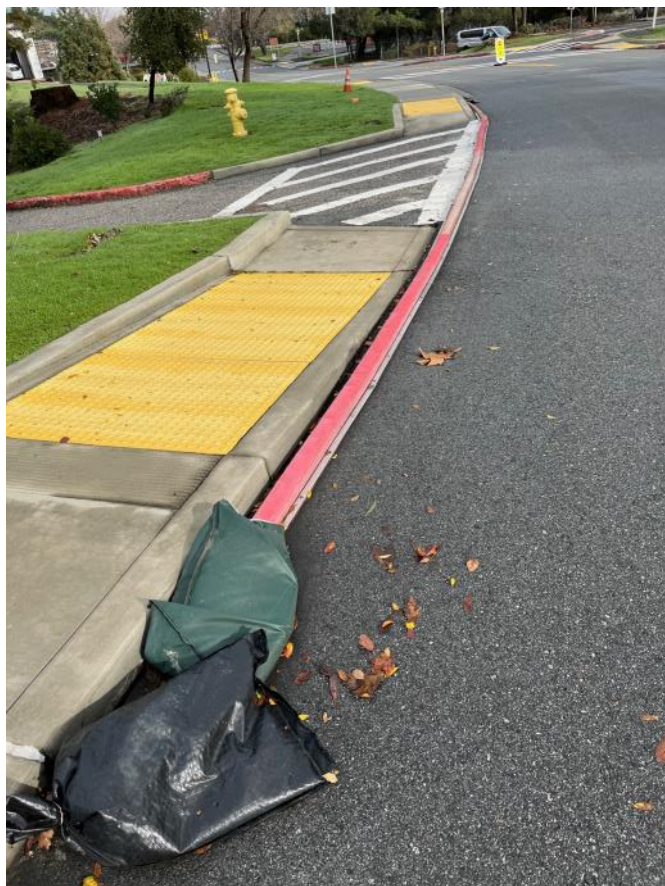
Figure 3. Spill containment berm used to divert water from driveway to basement.
